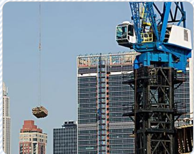
Construction materials and building 52
